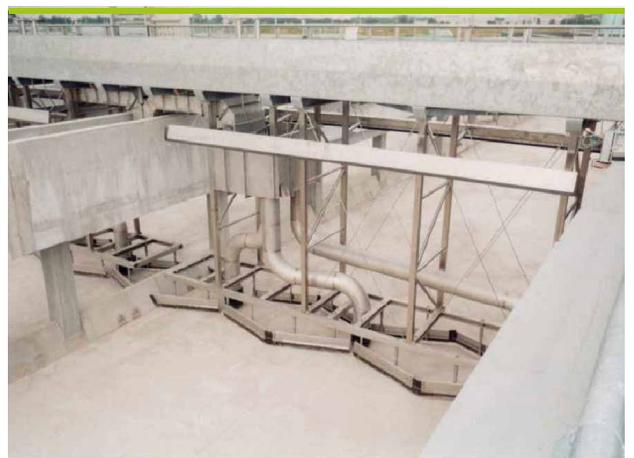
bottom scraping view with sludge collection by suction tube and sludge box – Milan WWTP (Italy)
