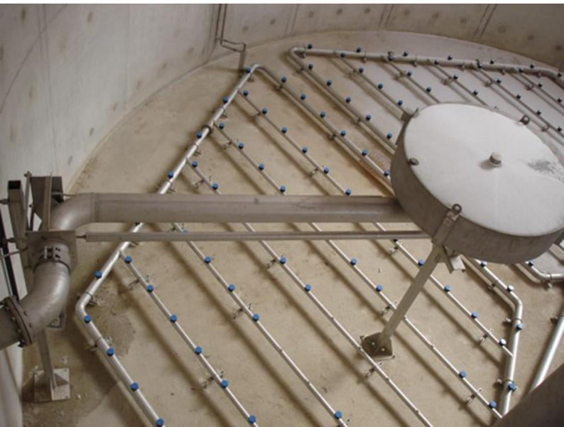
**The SBR (Sequencing Batch Reactor) process allows the completion of all treatment phases, successively, within the same tank**
