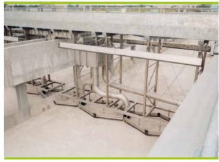
bottom scraping view with sludge collection by suction tube and sludge box – Milan WWTP (Italy)
