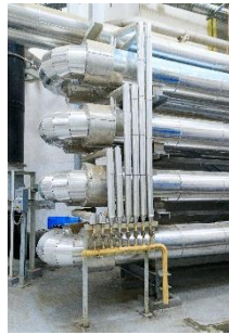
Digestion sludge recirculation and heating
