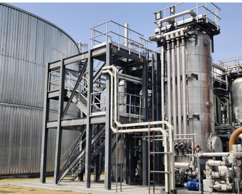
**Thermal hydrolysis disintegrates the cell structure of bacteria into an easily digestible and dewaterable product**
